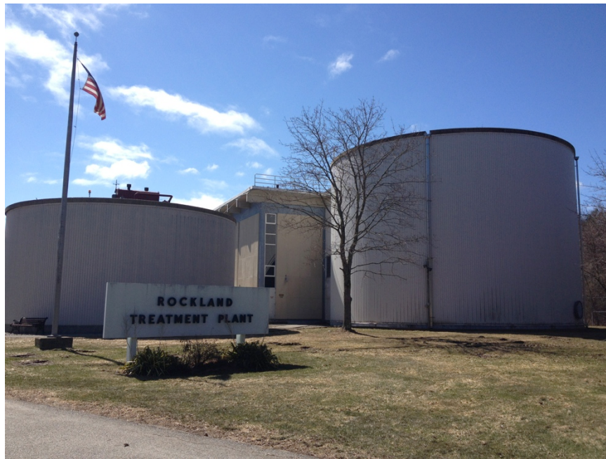
Figure 15: Rockland Wastewater Treatment Plant
