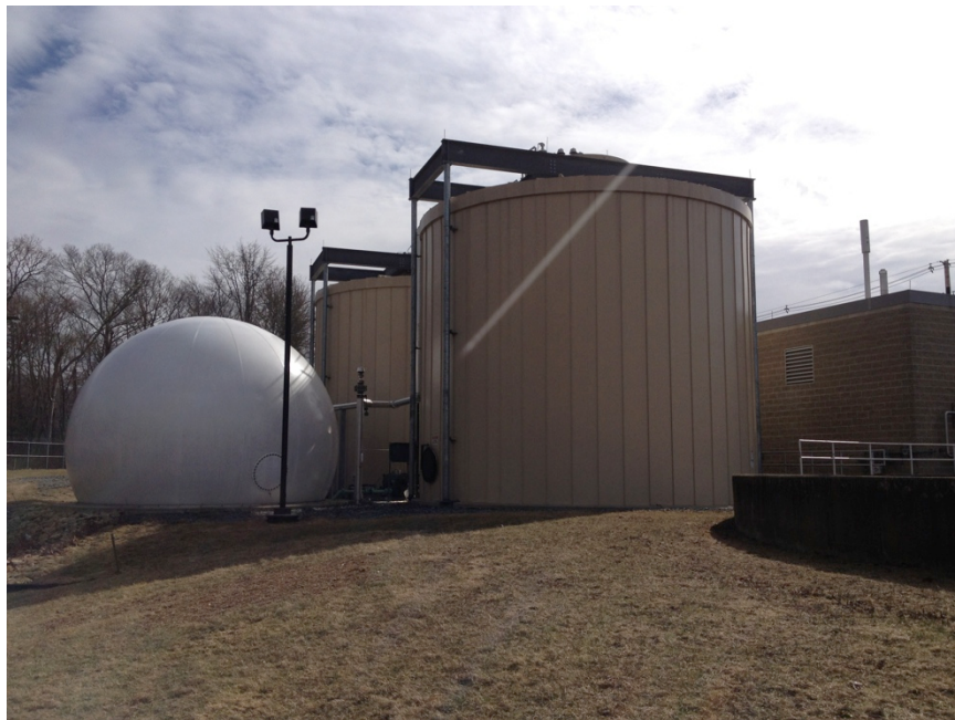
Figure 14: Fairhaven Wastewater Treatment Plant
