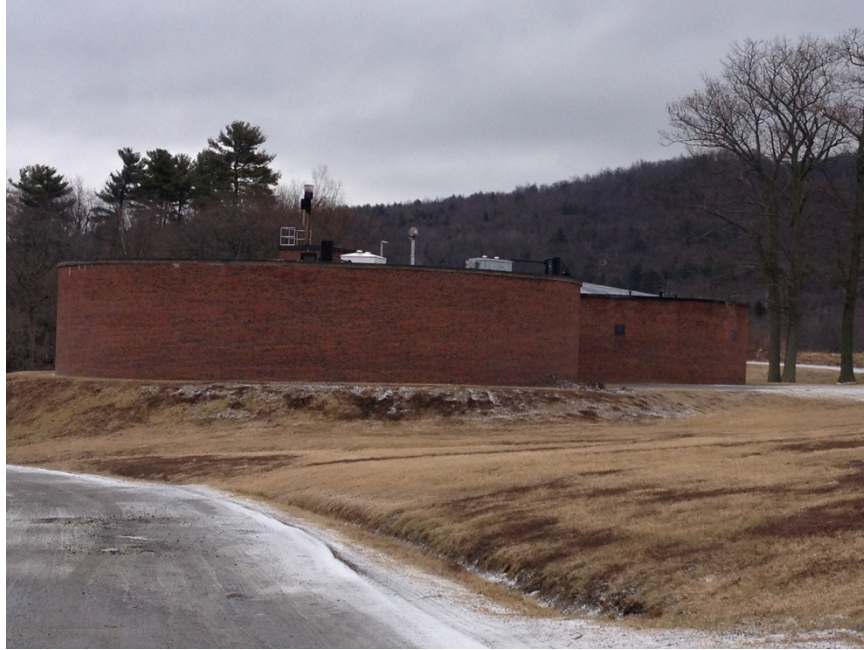
Figure 13: Pittsfield Wastewater Treatment Plant
