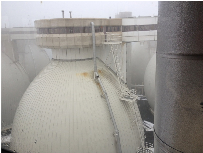
Figure 12: Deer Island Wastewater Treatment Plant
